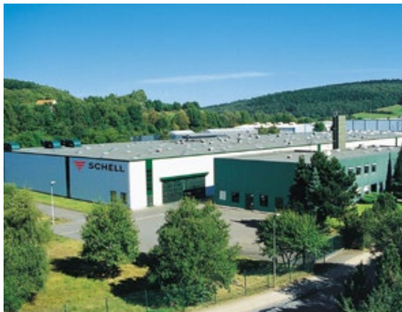
Plant 2 Production with logistics centre
